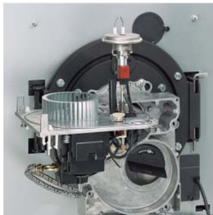
Fig. 25: Vitoflame 300 in maintenance position
