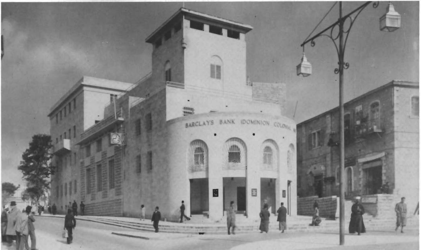
13. The New Municipal Building in Jerusalem, also occupied by Barclay's Bank. The building was usurped in 1948 by Jews.
